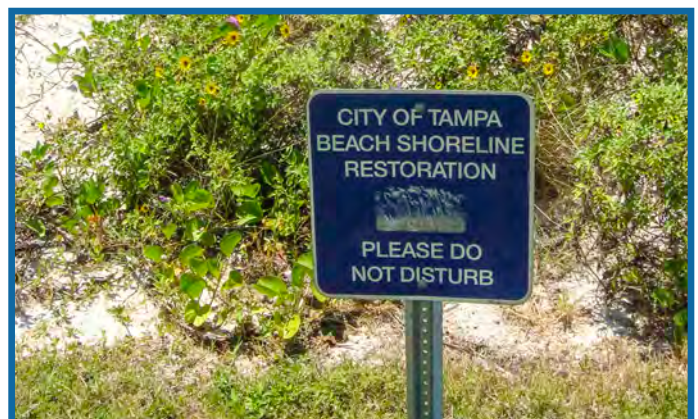
Man-Made Dune: A sand dune created by the City of Tampa on the Courtney Campbell Scenic Highway is helping stabilize the ever-eroding shoreline.
