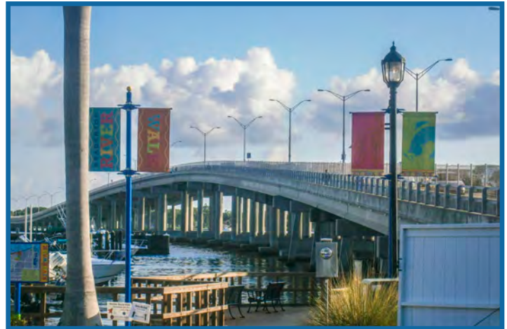
The City of Bradenton and Realize Bradenton lead efforts to install banner signs along the Tamiami Trail Scenic Highway to highlight events and attractions.
